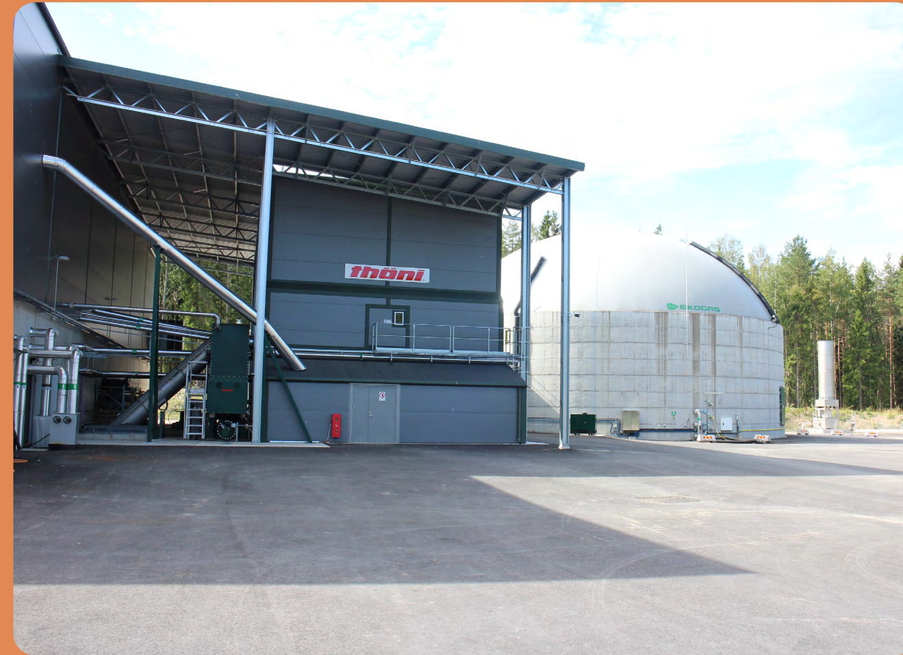
FIGURE 10: INTEGRATED HIGH-SOLIDS AD WITH IN-VESSEL COMPOSTING FACILITY IN FORSBACKA, SWEDEN
